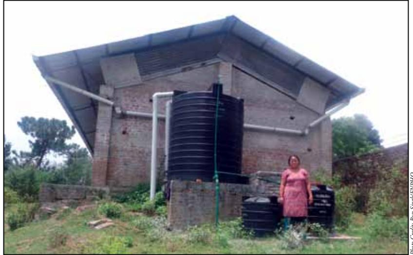
filtered water. The water is filtered through a Biosand Filter. Now, even when there is no tap water supply, the school can provide sufficient safe drinking water to more than 150 children and staff members. In addition, children do not have the burden of carrying water from home. Enough water to maintain their hygiene has provided an opportunity to live healthy, active and happy lives.
