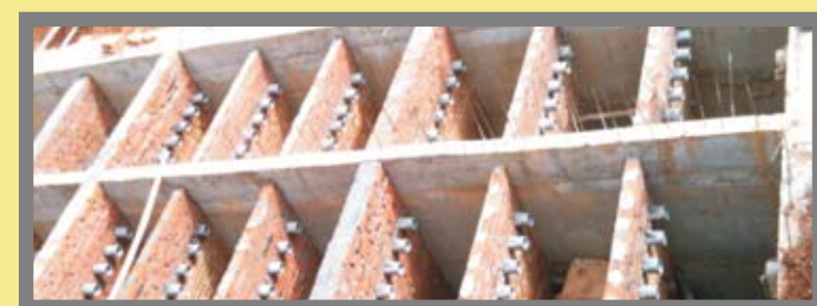
Anaerobic Baffled Reactor (ABR)
