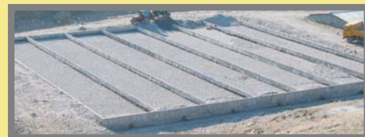
Sludge Drying Bed (SDB)
