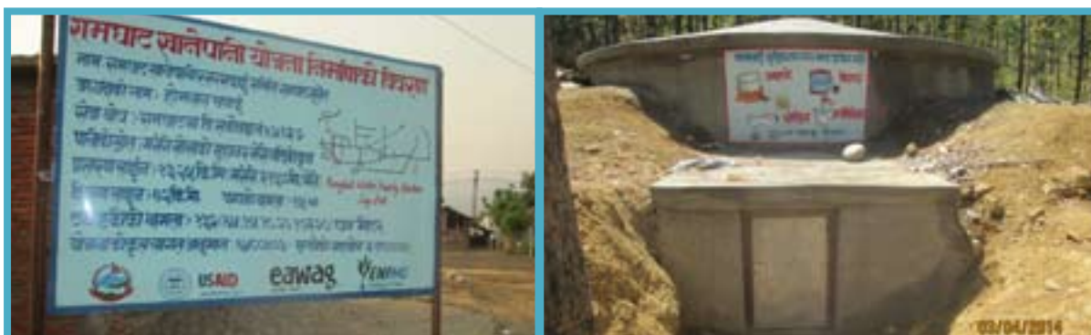
Ramghat Water Supply information board (left) and RVT tank installed (right)
