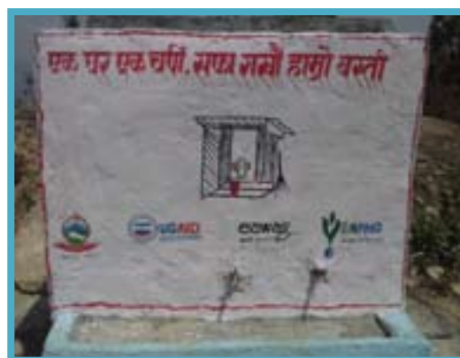
Water tank at Kaprichaur Sub-health post
