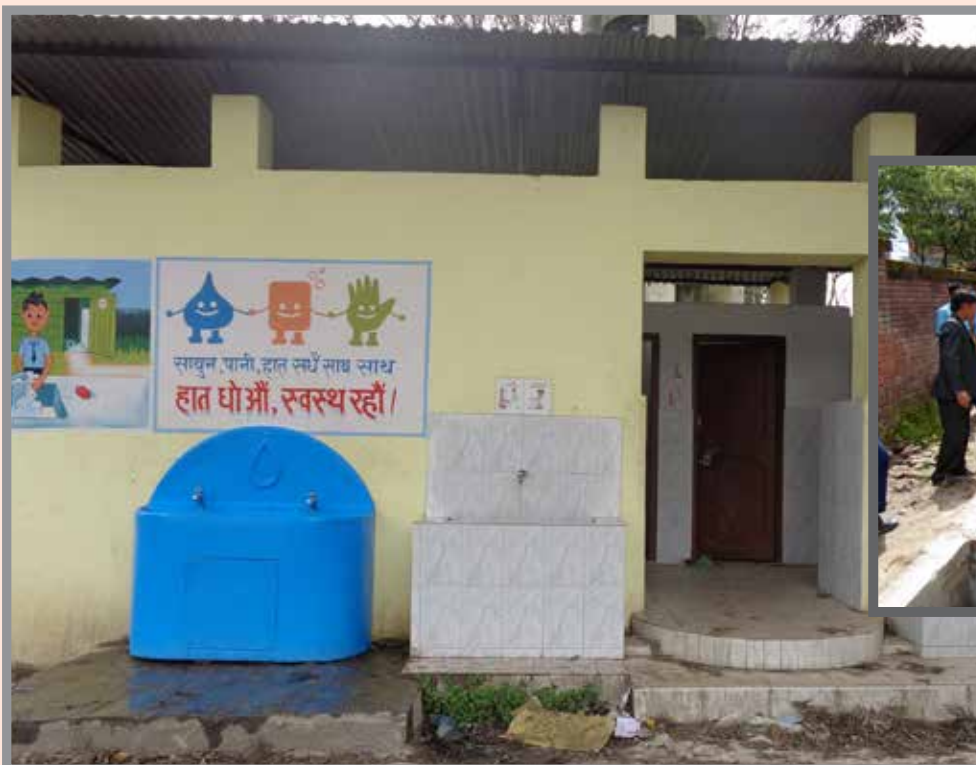
Construction of toilet
