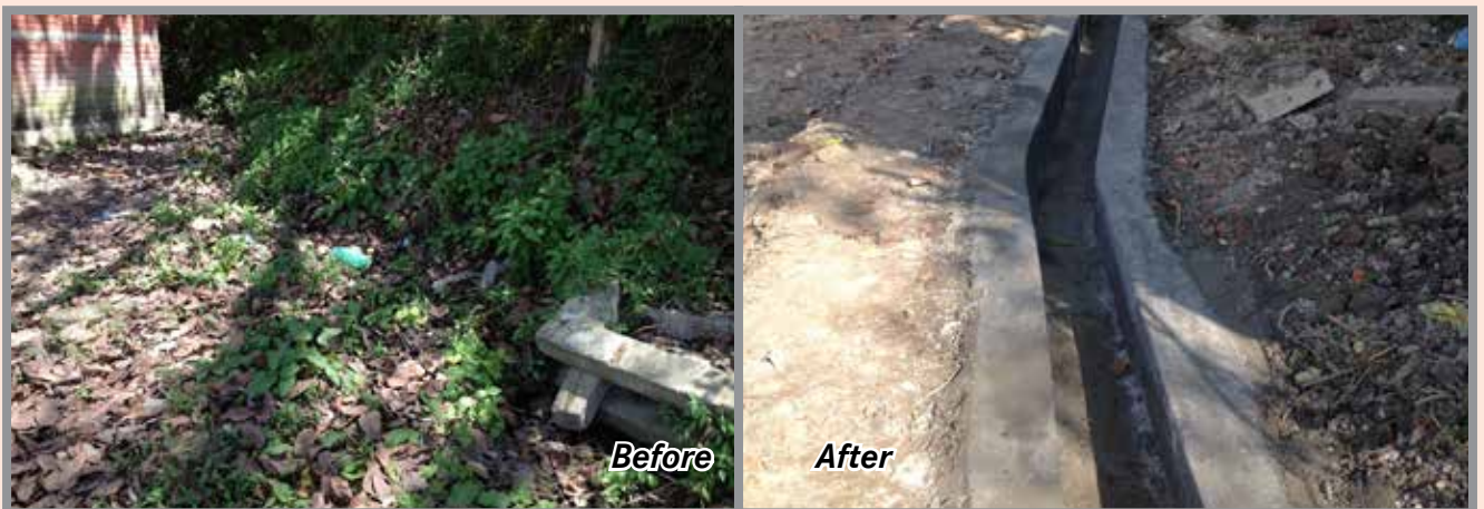
Construction of Drainage System at Shree Bal Premi Secondary School
