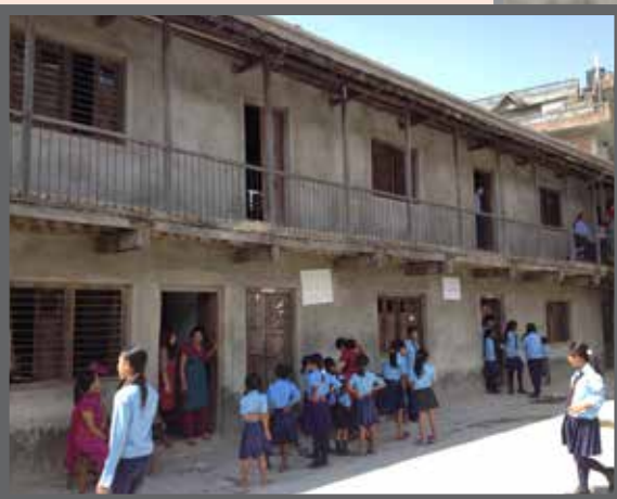
Plastering of school building
