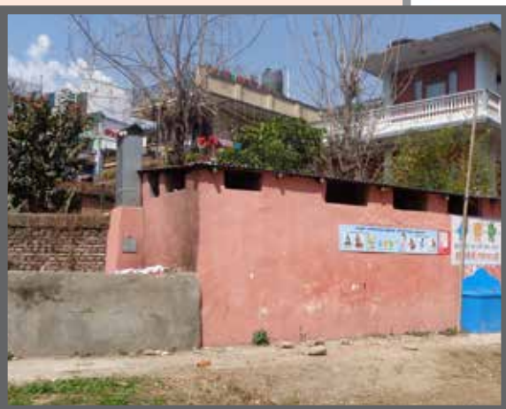
Construction of pad incinerator
