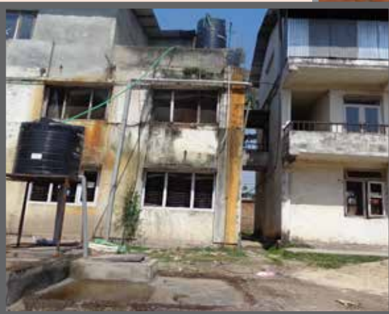
Installation of RWHS and construction of an underground tank
