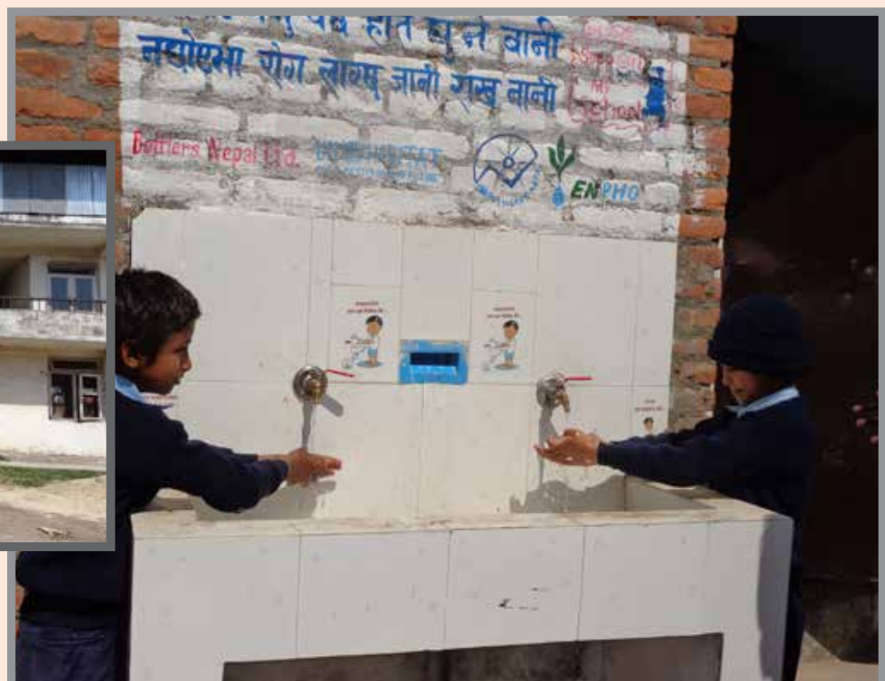
Construction of hand washing platform
