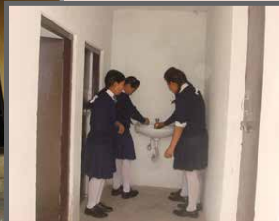
Construction of ladies' toilet
