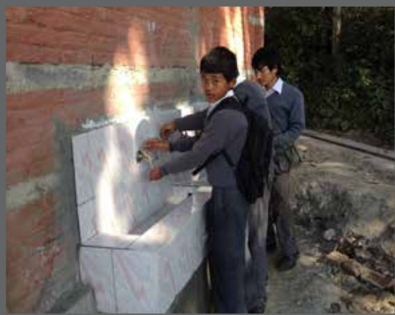
Construction of hand washing basin
