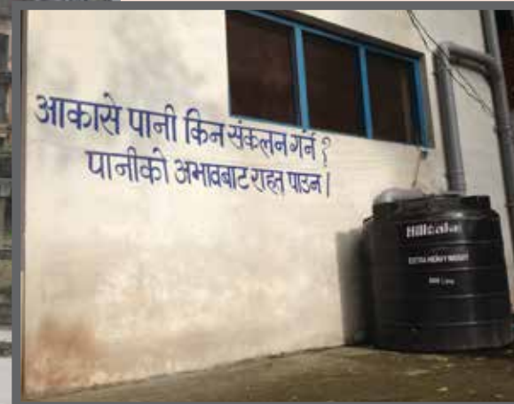
Installation of Rain Water Harvesting System
