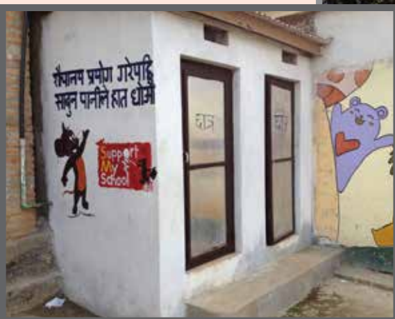
Construction of toilets
