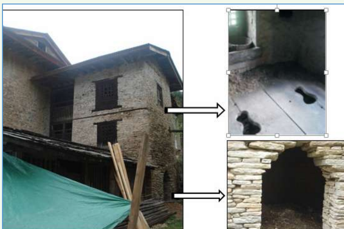
Traditional toilet of Sherpa community - Chasang built inside the house in Solukhumbu district
