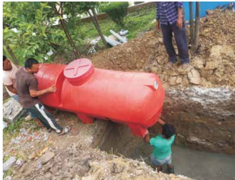
Installation of Septic Tank at Mahalaxmi Municipality
