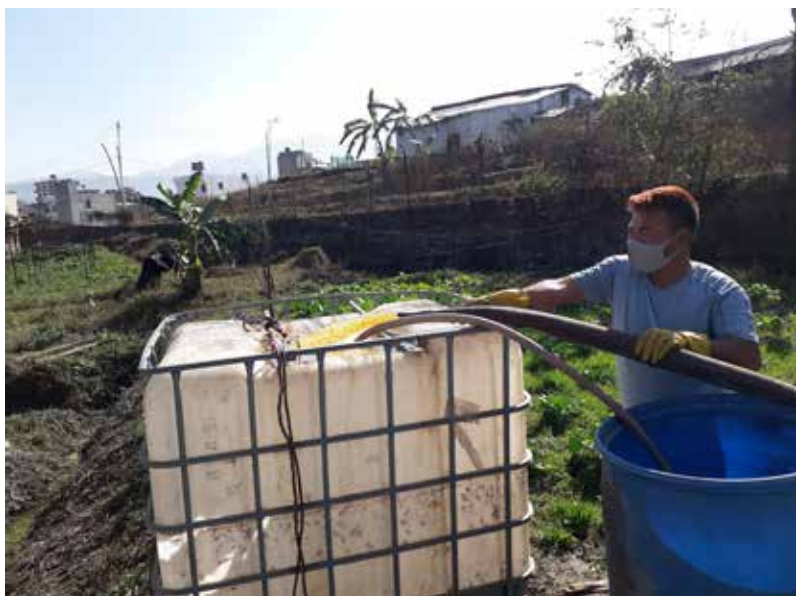
Faecal sludge from desludging vehicle being delivered to the experimental thickening tank
