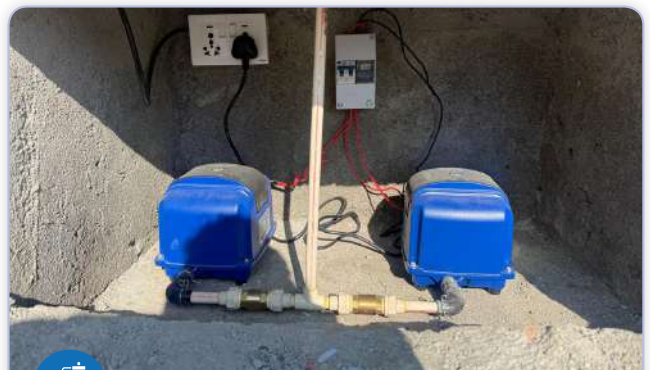
Air Pump for Wastewater Treatment Plant
